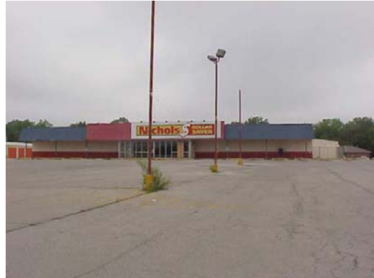
The old Nichols grocery store prior to renovations.
